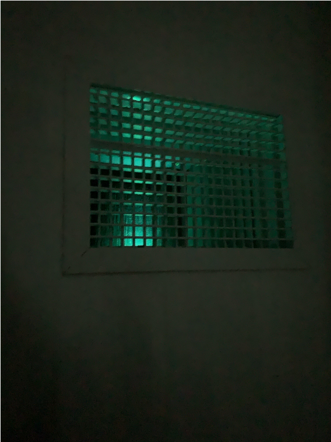
Photo 2 – FCU Installation (note green glow indicating cleaning is operative)
